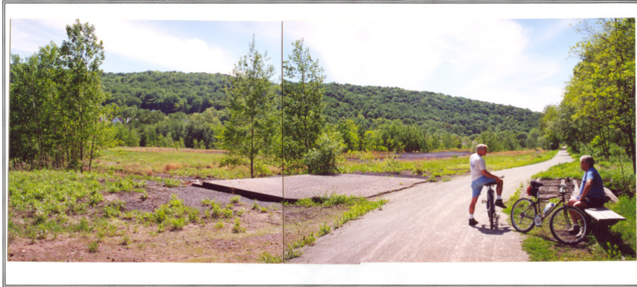
Exhibit 2.4 (H) Head of the Yellow Boy Channel at the Ghost Town Trail (under the platform and to the left). The old mine entrance is to the right. The platform is another historical remnant, which will stay as a reminder of the mining operation which was formerly the center of Vintondale.
