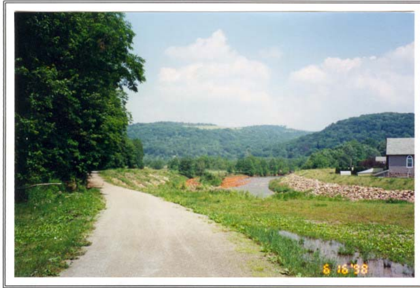
Exhibit 2.4 (B) Cross-section view looking east at the Bottleneck area. To the left is a steep hill covered by trees; in center is the Ghost Town Rail Trail, which edges a severe drop-off to the South Branch of Blacklick Creek. Notice how the rip-rap peters out on the left/north side of the creek bank.
