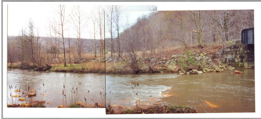
Exhibit 2.4 (M) Some rip-rap reinforces the project side of the South Branch of Blacklick Creek. This rip-rap begins at the Ghost Town Rail Trail bridge and ends before the Yellow Boy Channel downstream.
